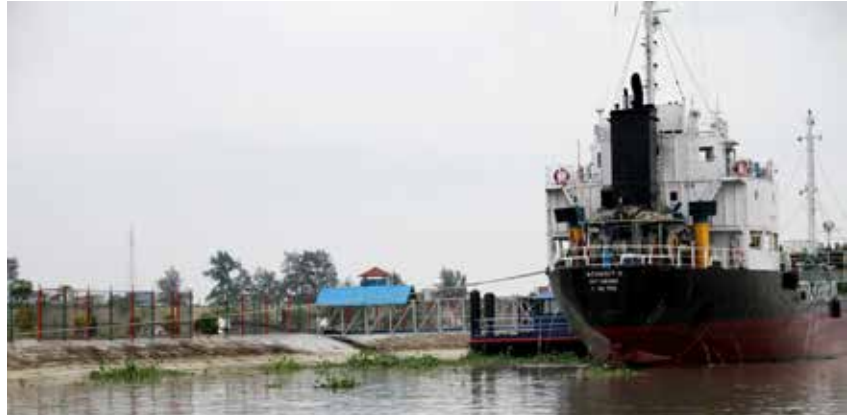
This 307 meter long river bank protection offers a good opportunity to reduce nearby in-stream erosion against the high flow
